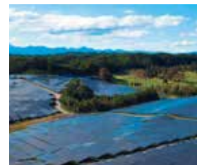
S-10 Takasaki Solar Power Plant A
