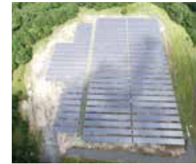
S-02 Chiyoda Kogen Solar Power Plant
