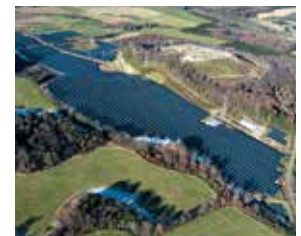
S-09 Monbetsu Solar Power Plant
