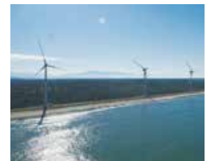
W-01 Tainai Wind Power Plant
